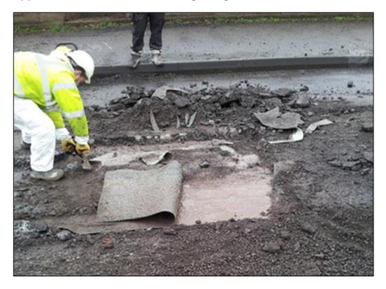
1. Failure of waterproofing due to lack of bond with deck concrete
