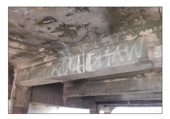
3. Leakage through deck and ongoing deterioration of repaired areas
