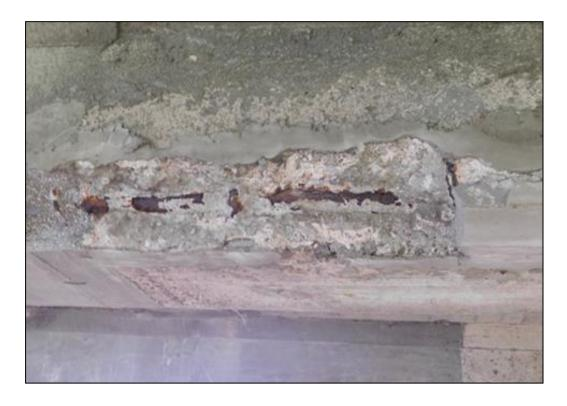
2. Failure of previous repair due to continuing corrosion of reinforcement
