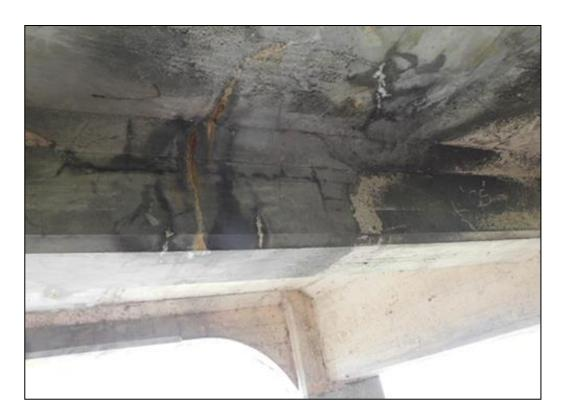
4. Leakage through deck and ongoing deterioration of reinforced concrete members
